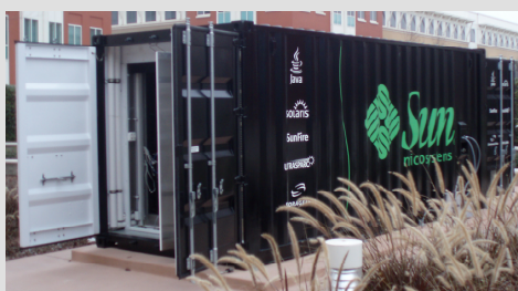
A Sun server-packed container designed for rapid data center deployment (source: J. Gallagher)
